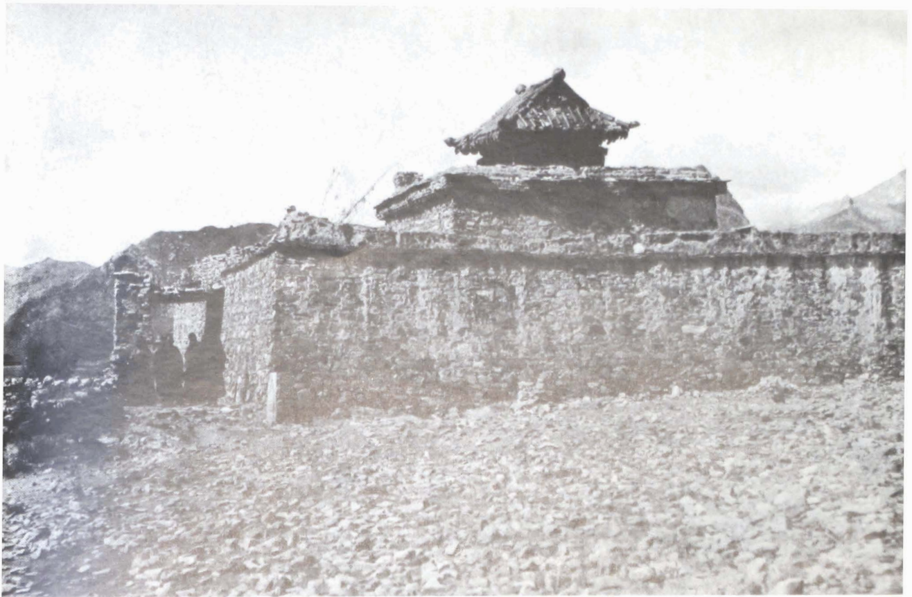
(above) Tomb of rNgog Blo-ldan shes-rab (eleventh century). An early example of a tiled pagoda-style roof combined with normal Tibetan building (see pages 141 and 160)
